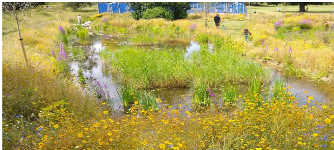
Example of the wetlands Enfield Council built in Enfield Town Park 2018 which helps to store and treat water before it enters a watercourse. Also creating an attractive place to visit
